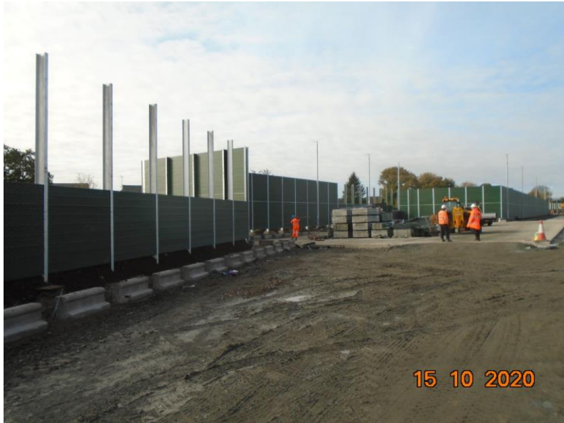
Kerbing / Pre-Surfacing / Fencing Works
