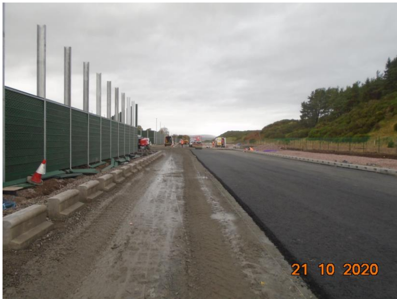
Surfacing / Fencing Works
